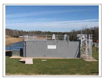
either above grade, as shown, or below grade. Not shown in this picture are the other process units such as the clarifier, sludge holding, and any tertiary of disinfection.
