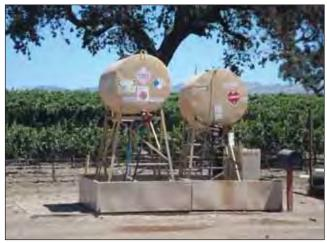
**PHOTO 10:** View of gasoline, diesel and waste oil storage containers.
